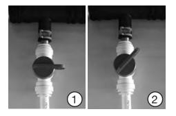
The flow control and thus the efficiency of the two water circuits (living room/bedroom) can be regulated by means of the shutoff valves.
